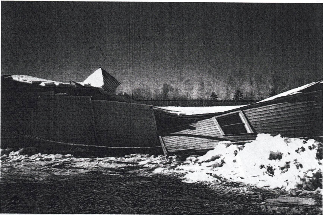
Town Hall Collapse -Two views (side and back) of damage to the Industry Town Hall from the weight of snow and ice. Feb. 11, 1998.
