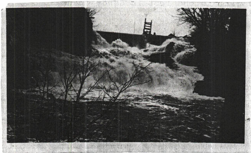
This photo offers a close-up view of a dam on a brook running through West Mills.
