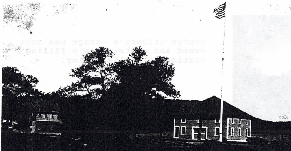
Left: This lakeside view shows both the garage (right) and the grange hall (left).
